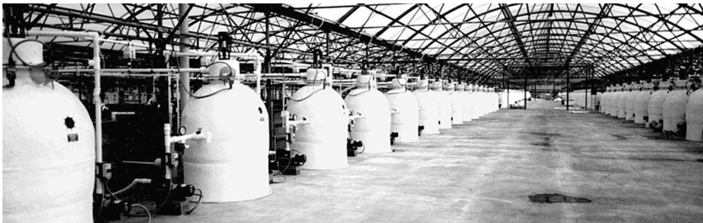
An example of floating bed filters used as bioclarifiers in a large indoor tilapia grow-out facility in the midwestern United States. Photo supplied by Aquaculture Systems Technologies, LLC.
