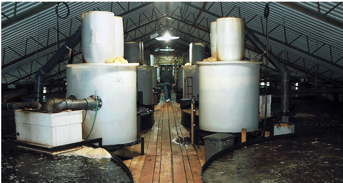
Eastern Tilapia's recirculation system features growout tanks with packed columns, biofilters, and low-head oxygenators.
