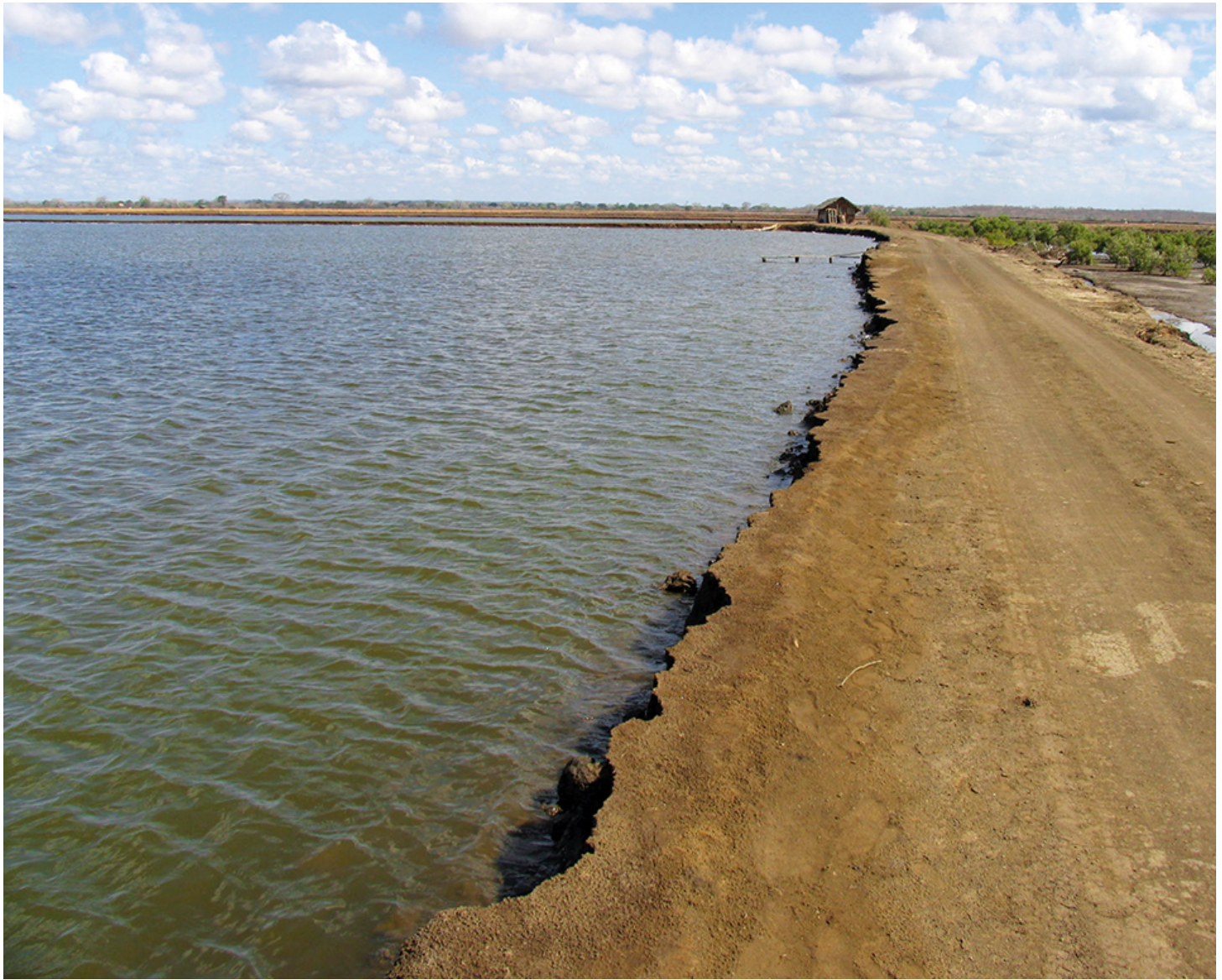
Improper construction techniques can lead to erosion of pond and canal banks.
