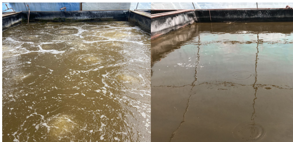
View of tanks with an activated aeration system (left) and without an aeration system (right).
