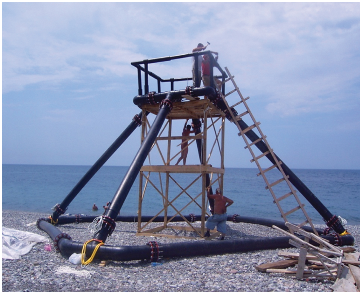
An OCAT cage constructed on the shore of the Black Sea was towed offshore and stocked with trout fingerlings.
