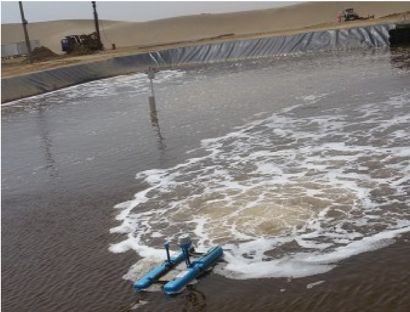
Each trial pond had aerators at opposite sides to create a smooth water current flow, maintain dissolved oxygen levels and accumulate sludge in the center for removal.
