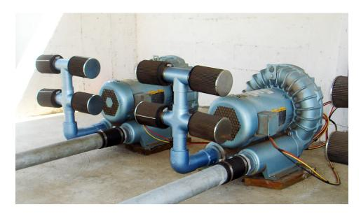
The use of large-diameter plumbing minimizes friction losses in regenerative blower systems. Inlet filters protect the blowers and air distribution system from dust and other contaminants.
