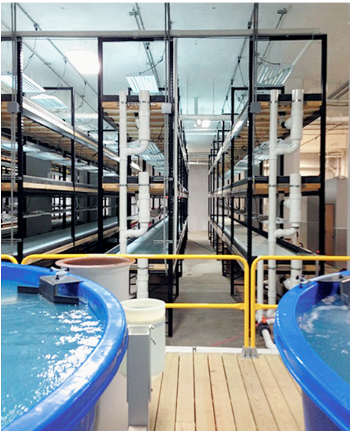
At the Hamm's Brewery project, fish culture tanks recirculate water with three-tiered racks of plant-growing trays.
