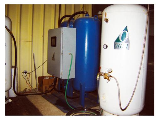
This oxygen generator and its oxygen storage cylinder employ highpressure swing adsorption to produce oxygen.
