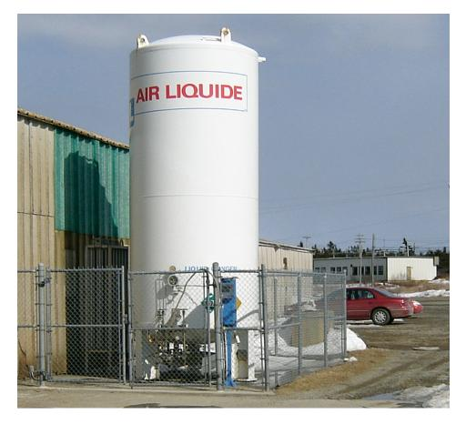
Liquid oxygen is normally trucked in and stored in a bulk tank in liquid form.
