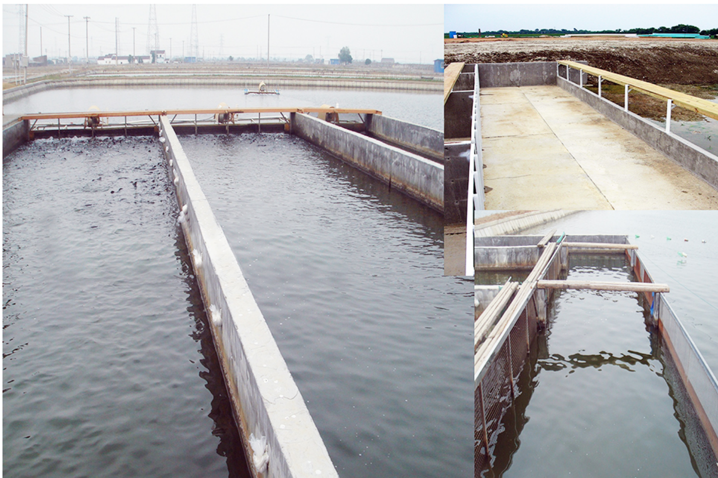
At the intensive pond aquaculture demonstration site, raceways are positioned within the pond for fed fish (left). Waste collects in the quiescent zone at the end of the raceways (right).
