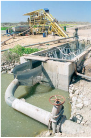
Some reservoirs have concrete harvest pits with strainers for separating the fish from the water as well as life-support features to ensure the welfare of the fish. Photo by David Jansen, Visible Voices Media, Israel.
