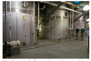
New large-scale fermenting equipment with automated controls and monitoring will support microalgae product and process development.
