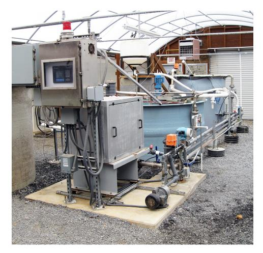
The membrane biological reactor located at the Conservation Fund's Freshwater Institute was operated for the recovery of not only water but alkalinity, salts, phosphorus and protein.
