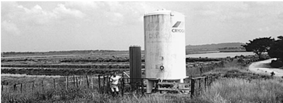
A cryogenic liquid oxygen tank stores oxygen for the system.
