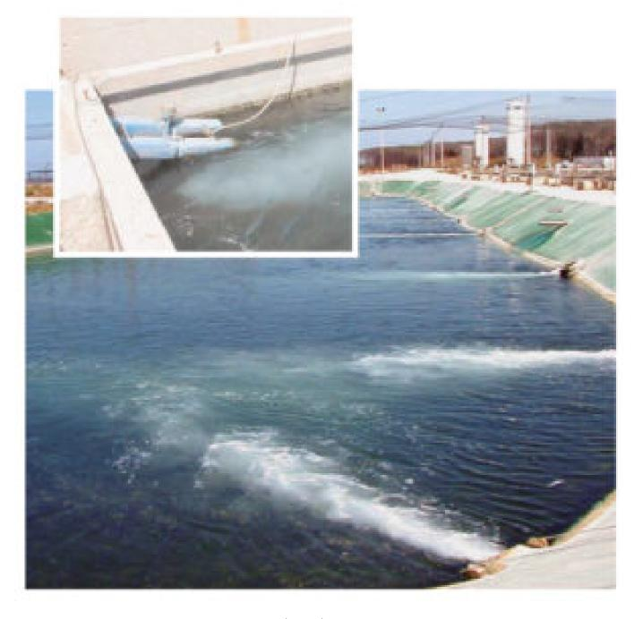
Force 7 aerators inject oxygen into raceways (above). Both source water and culture water receive oxygen injection to raise oxygen levels.
