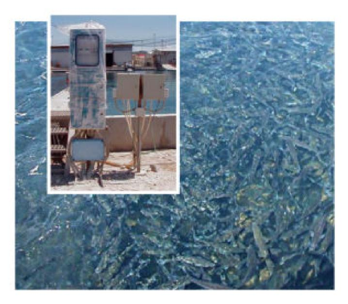
Each raceway has a computerized control panel that monitors temperature and dissolved-oxygen levels to maintain optimum conditions for the cultured fish.
