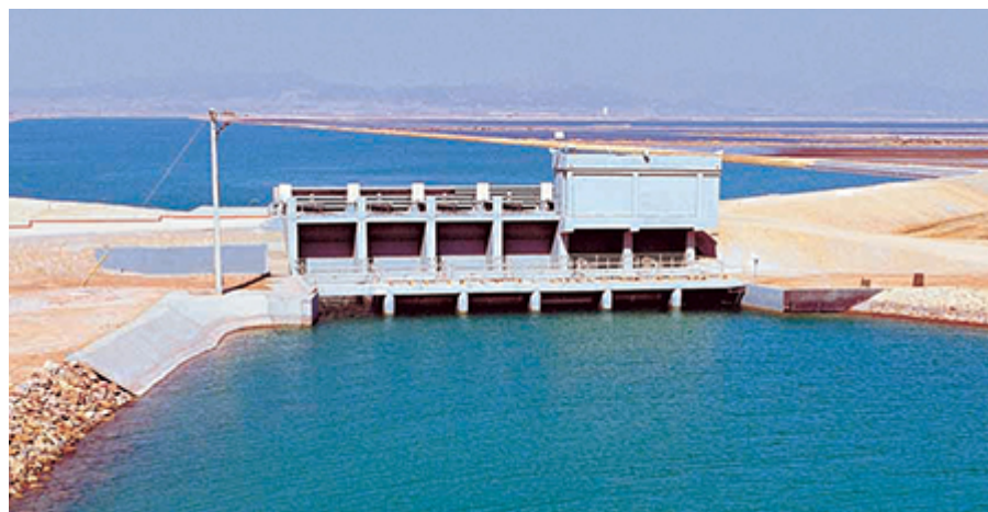
Pumping stations move water through a 38-km canal system.
