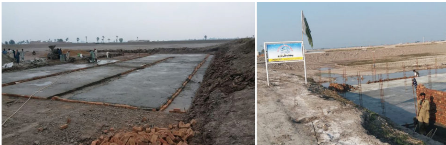
Views of the construction of the first in-pond raceway system (IPRS) technology demonstration site in Pakistan, showing the floors of the raceways, concrete pillars and raceways walls.
