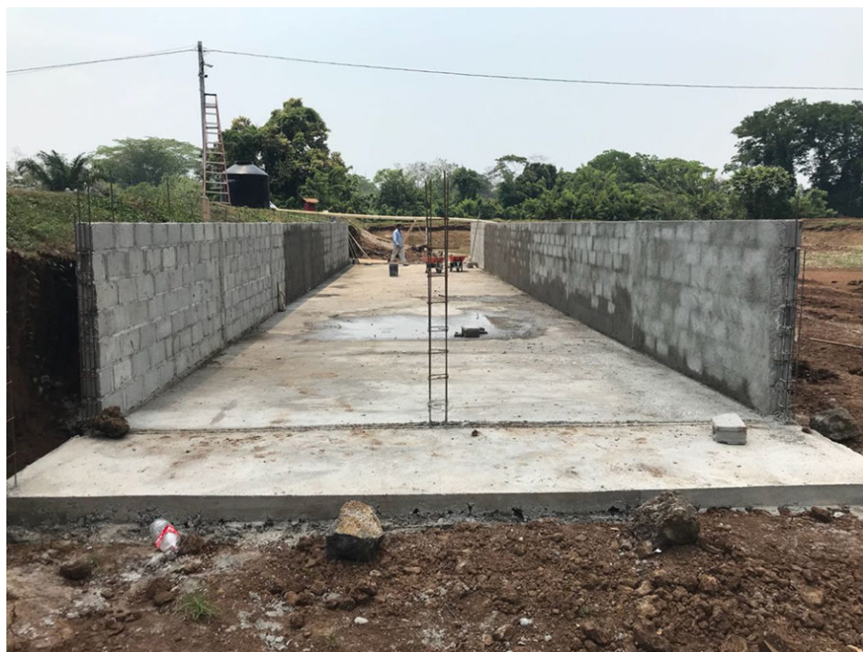
View of the demonstration in-pond raceway during construction. Note the fixed, cement floor on the pond bottom.
