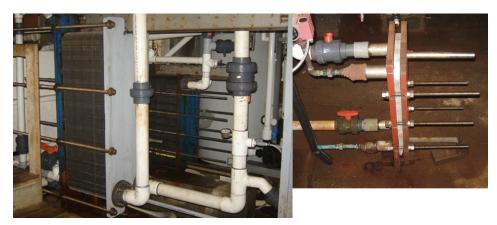
Properly sized water-to-water heat exchangers should perform at greater than 90 percent efficiency.
