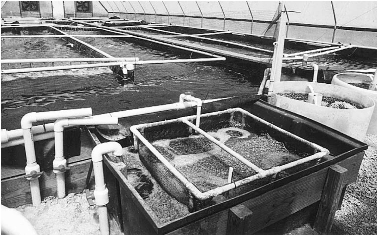
The filtration system in shrimp recirculating raceways at Harbor Branch Oceanographic Institution (Fort Pierce, Florida, USA) uses a nitrifying biofilter to convert toxic ammonia to non-toxic nitrate. Photo by Darryl E. Jory.
