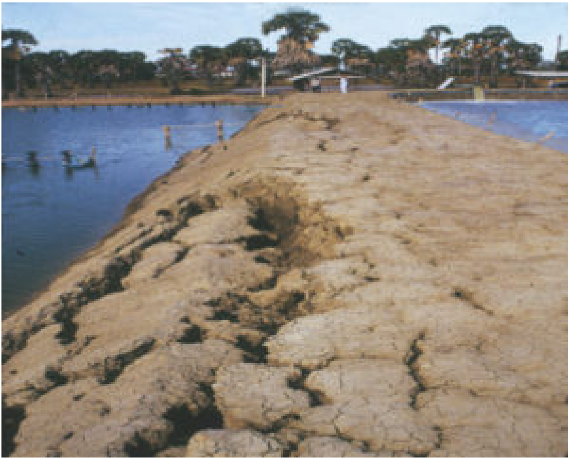
Embankments made of heavy clay soils must have adequate side slopes or they will slip.
