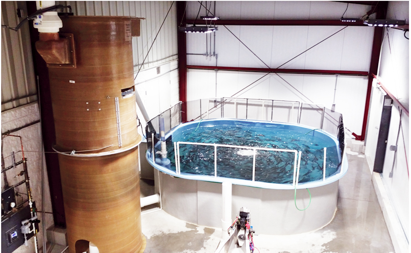
The Freshwater Institute's purge system utilizes partial water reuse without a biofilter.
