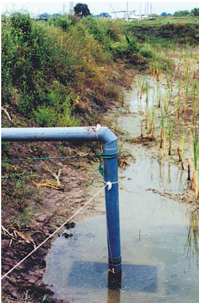
Sump pump for water reuse after passage through sedimentation pond and artificial wetlands.
