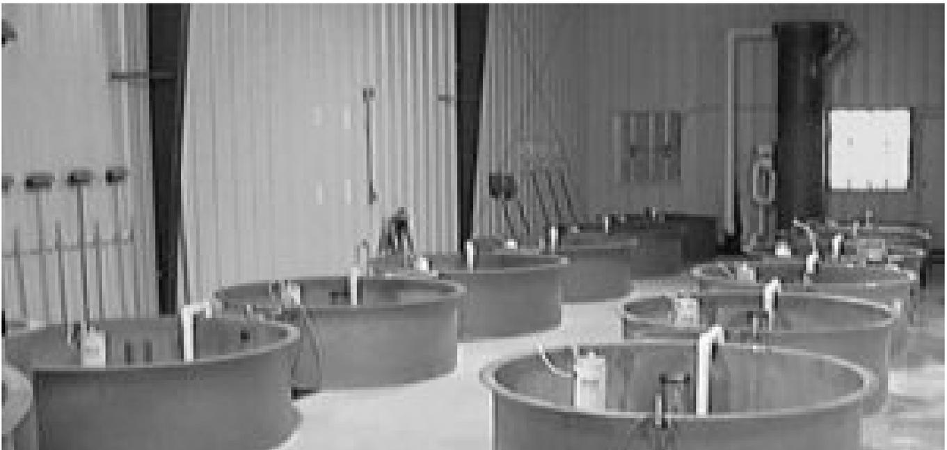
Before water enters the fry tanks, a nonpressurized packed oxygen column (behind culture tanks in this picture) adds pure oxygen to the water while driving out dissolved nitrogen.
