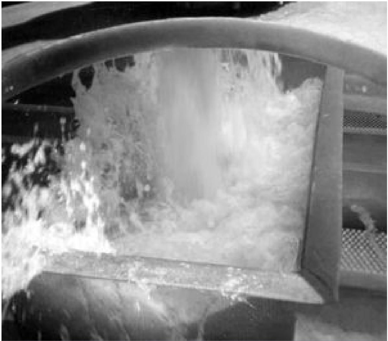
Water is broken into droplets as it flows through a counter-current forced-air cascade stripping column installed in the top portion of a water reservoir tank at the MCRA Hatchery.
