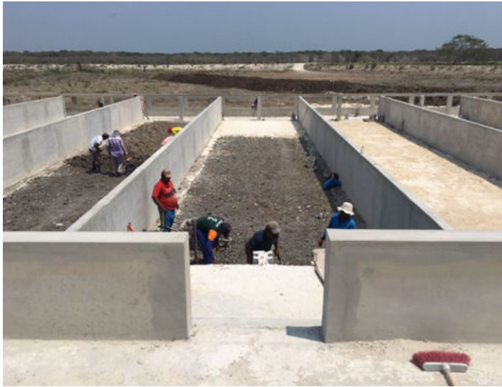
View of raceway construction for the demonstration project.
