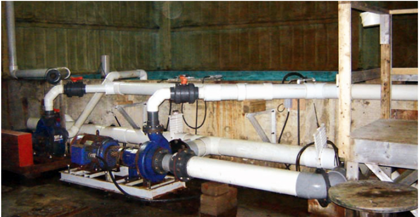
Properly configured supply pipes provide the unobstructed water flow that helps limit cavitation.
