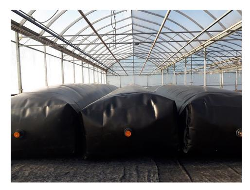
The Sth'oqui Aquaculture Limited Partnership of the Sumas First Nation, which operates a 100-metric-ton tilapia farm in Chilliwack, British Columbia, now uses an anaerobic digester that converts fish waste to biogas, which is stored in these bags.
