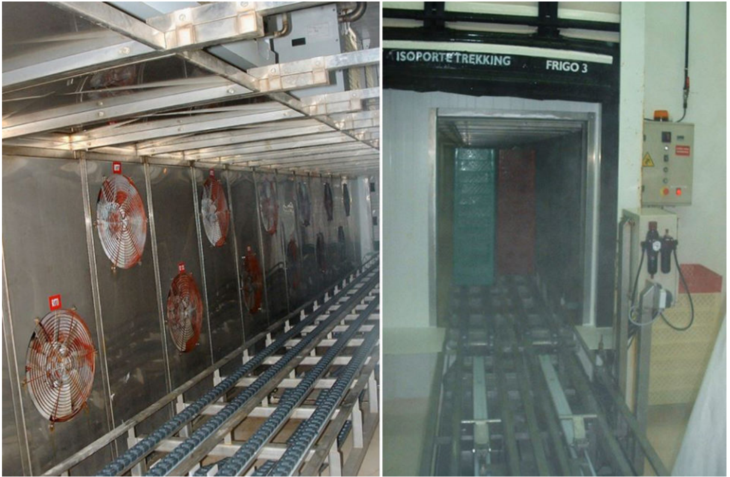
Views of air blast tunnel: inside an air blast tunnel (left); and piles of shrimp blocks going into the tunnel (right).
