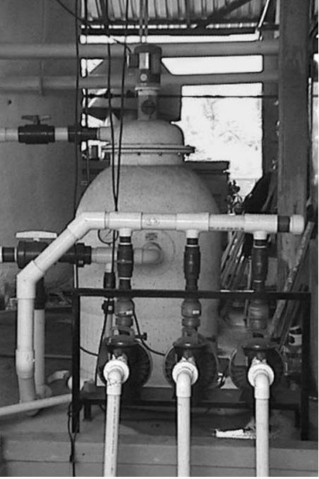
Pumps supply recirculated water into a fluidized bed biofilter at Maricultura del Pacificio.
