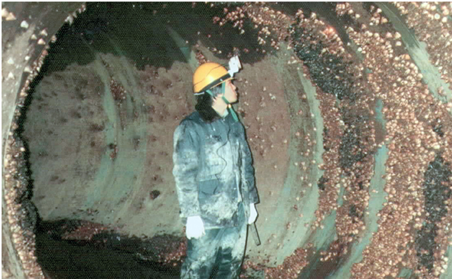
Mussels attach to and grow on the surfaces of power plant water intake pipes.
