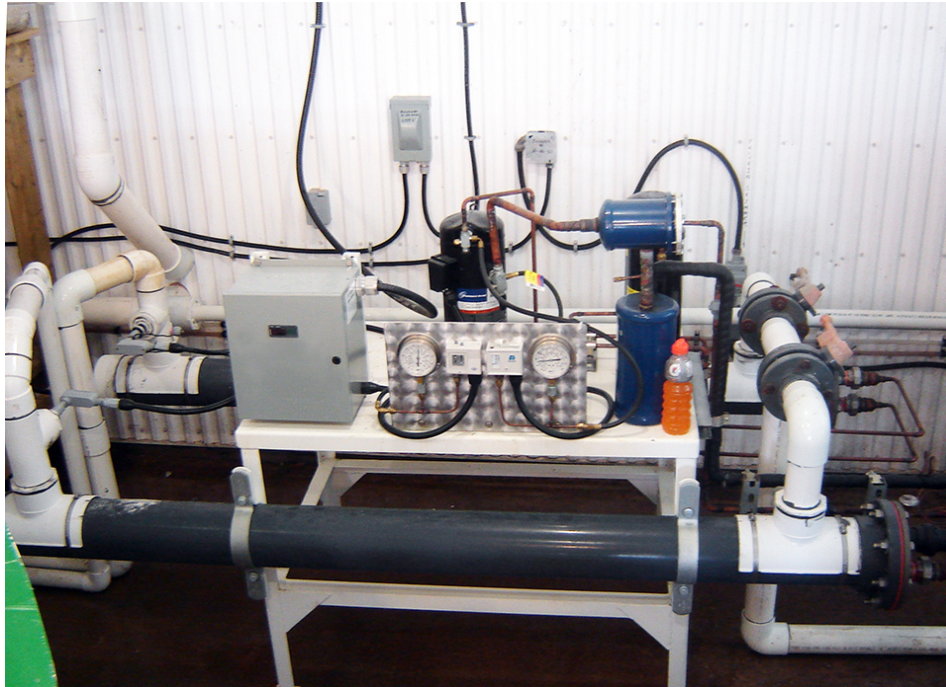
This custom-built water-source heat pump has a COP over 4.5.
