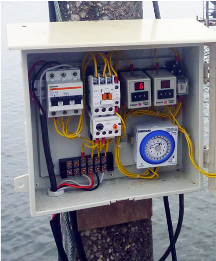
In small culture ponds, an automatic feeder can broadcast feed in a radius of 10 m and feed 600,000 shrimp. Timers control the broadcasting times and intervals of feeding.
