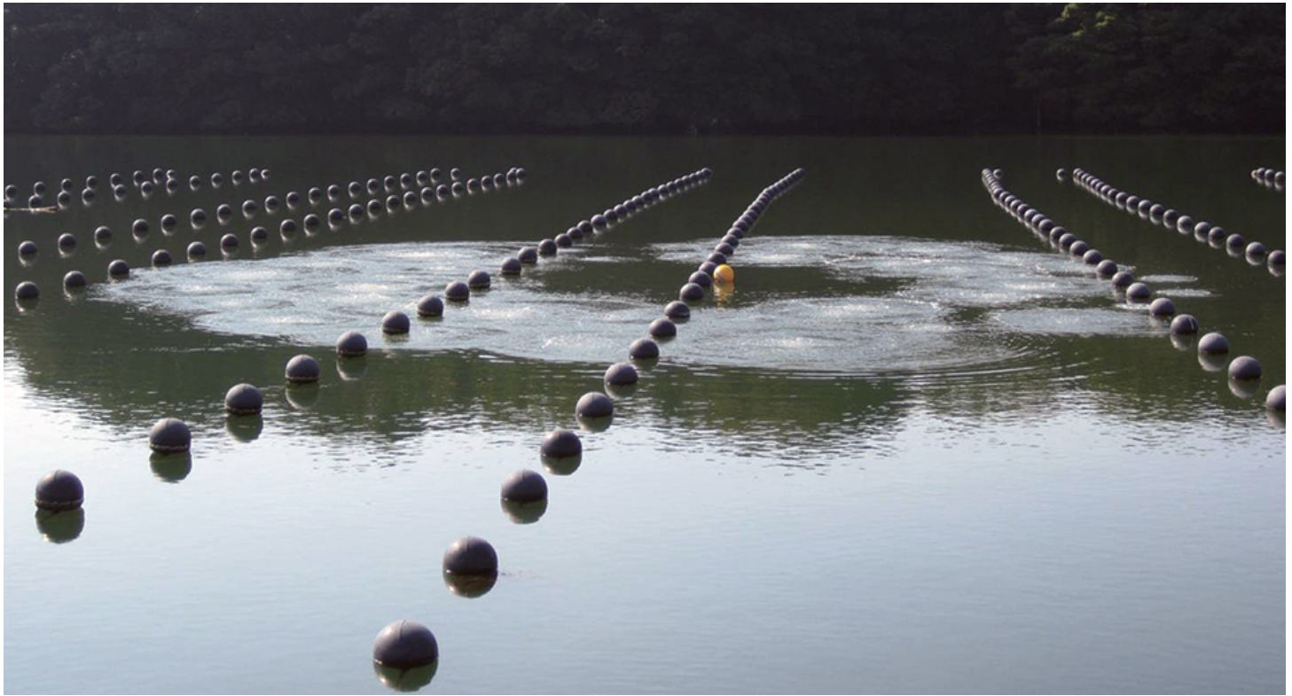
A circular configuration of tubing pumped water up from the lower depths of the bay, resulting in waves on the surface. The aeration center is located at the yellow buoy.
