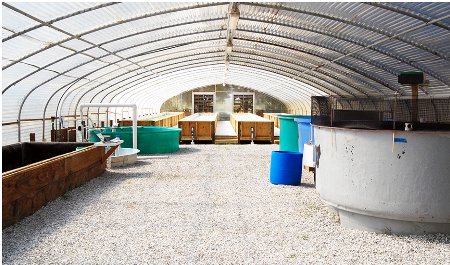
Water from the plant raceways in the rear of this photo is pumped, filtered and reused in the fish culture tanks (right foreground.)
