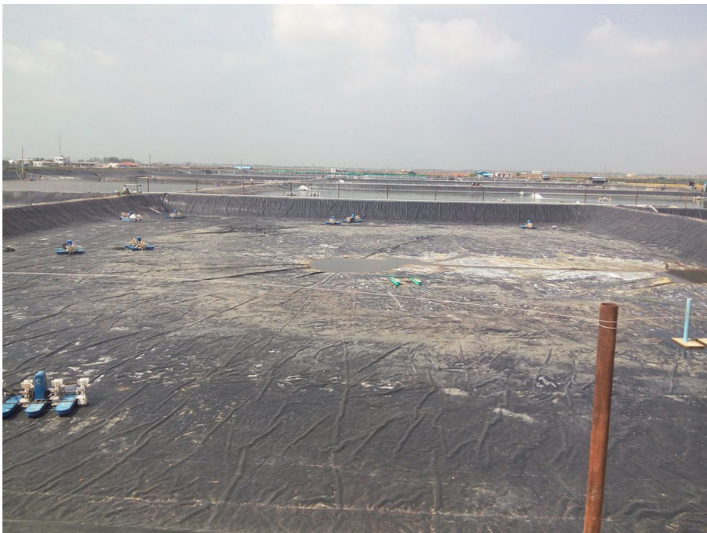
Lined shrimp ponds that are well-designed, built and managed can efficiently manage organic matter and sludge. Note central drain and accumulated sludge in center of pond. Photo by Amit Ranjan.
