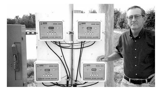
Mississippi (USA) grower Chip Otts uses automated monitoring to remotely and effectively – manage his five catfish ponds.
