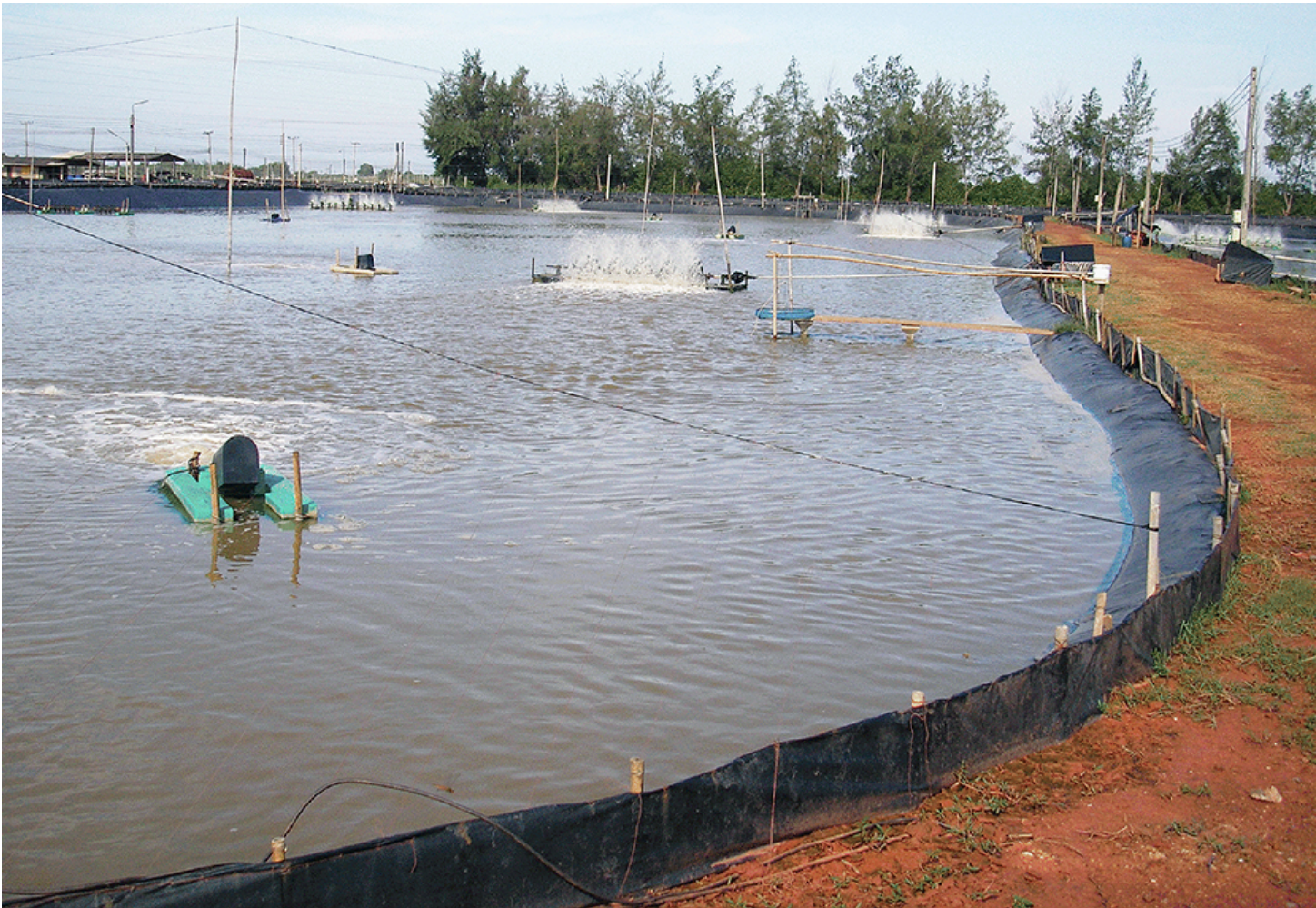
C.P.'s lined ponds include biosecurity barriers to exclude pathogen carriers and mechanical aeratorsto improve oxygen levels and maintain bottom conditions.
