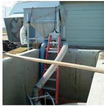
Previous manual harvesting of raceways has been replaced by a more automated system using a harvest basin, fish pump and dewatering device.
